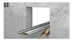
Clean the aperture and remove all loose parts. Check the correct installation of the cable tray/ladder on wall and floor. Cable trays and ladders shall be supported 250 mm and 500 mm apart from walls and  $\leq 550$  mm above floors.
